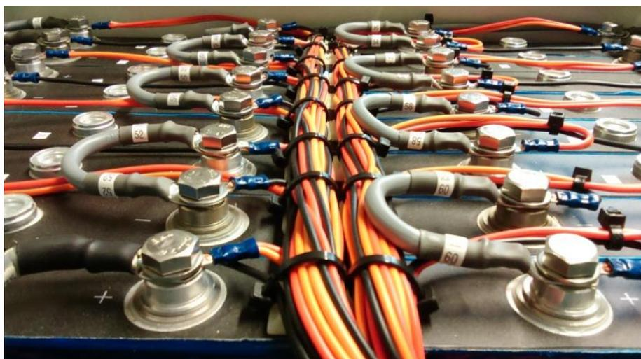
Fig.2 LiFePO<sub>4</sub> storage system connections.
